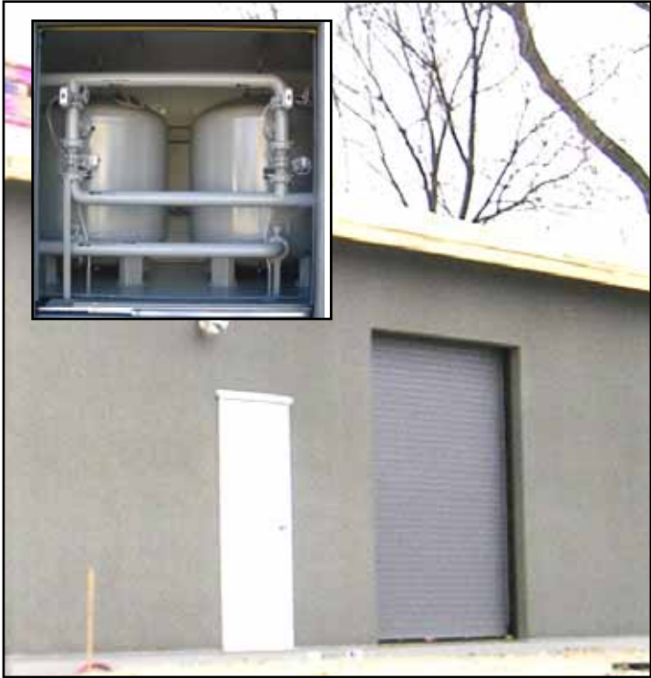
Here shown is the the man-door and overhead door in the eastern building half for access to the 4500 gallon detention tank and two 7 foot diameter pressure filter tanks with filter controls.
