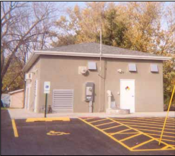
Here shown is the the finished installation with the roof complete, the fascia, soffits, gutters, downspouts, and seam strips attached. The three doors, rear to front, are the pre-treatment chlorine feed room, the office and control room, and the stand-by generator room to the front.
