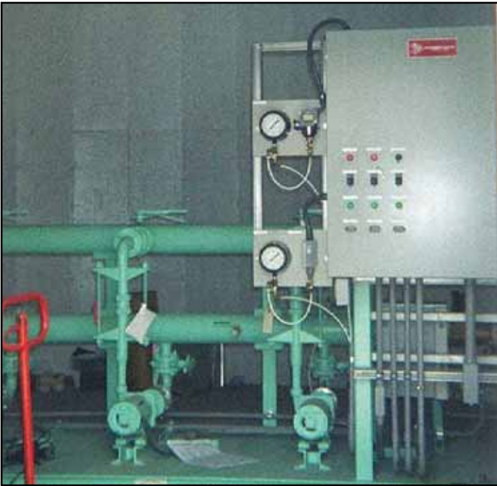
Here shown is a view into the elevated tank base showing the skid, tri-plex booster station and pump controls.
