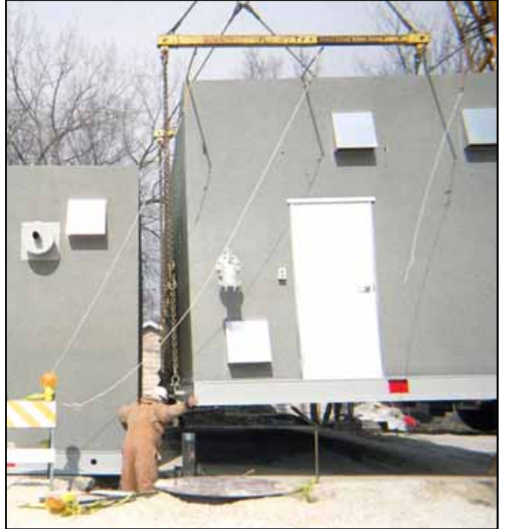
Here shown is the eastern half of the building being guided into its final location.
