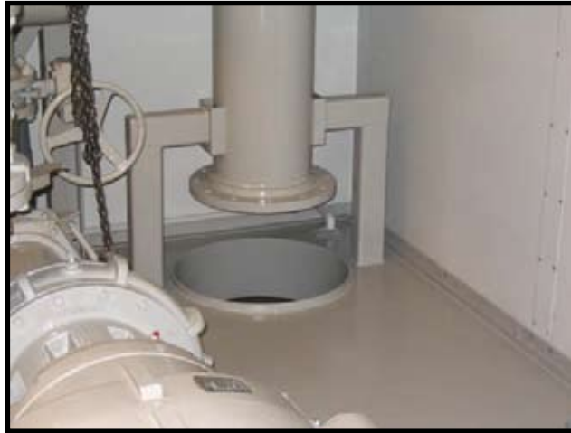
The installing contractor makes inlet and outlet connections.
