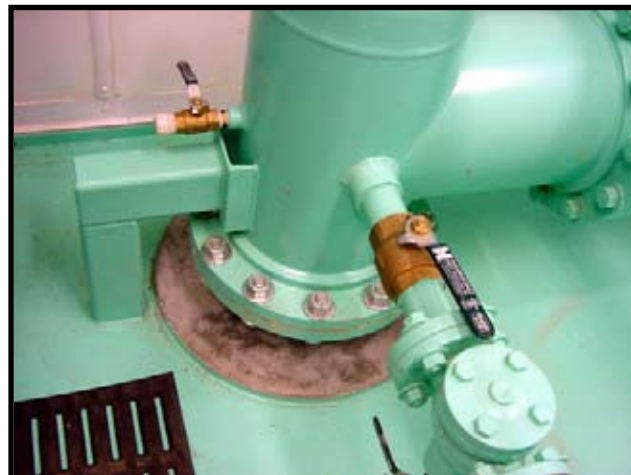
The pipe has been grouted to the sleeve, sealing the station.
