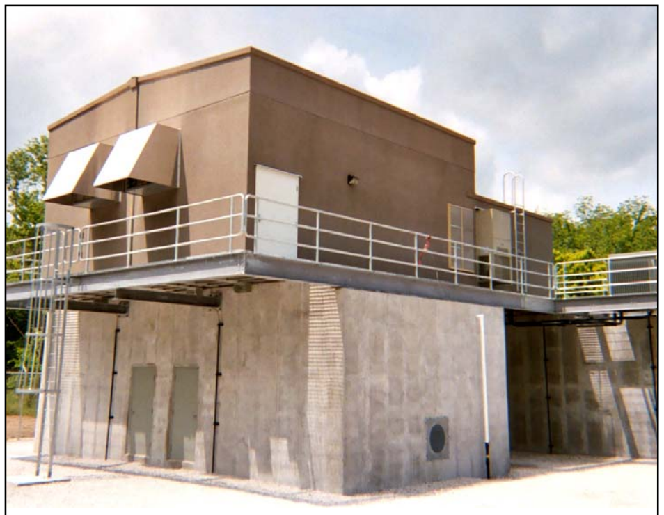
Completed Raw Water Pump Station with intake structure.
