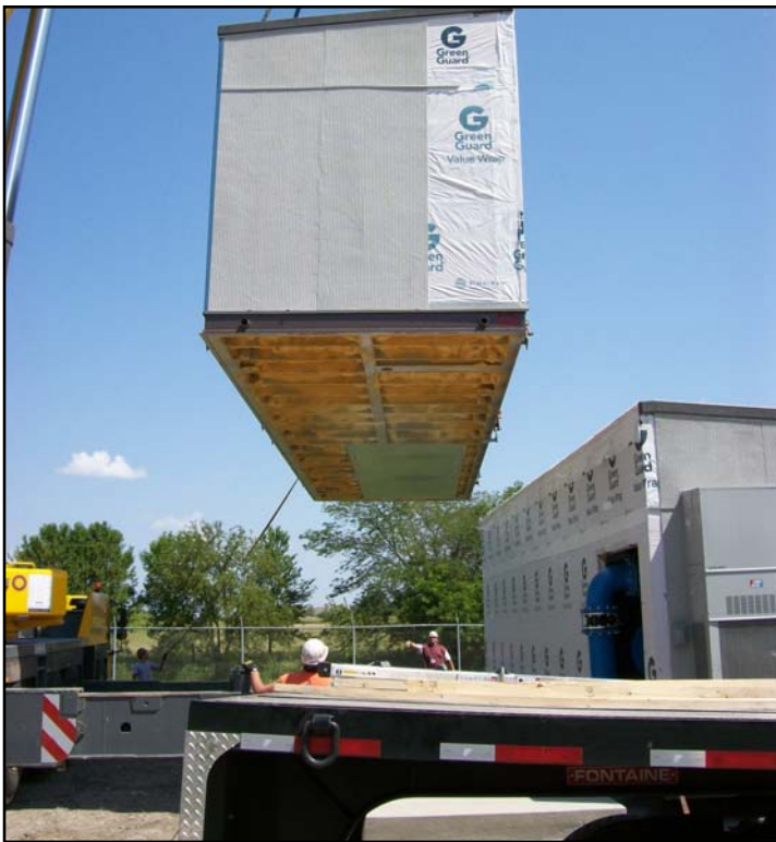
This project in Iowa is being off-loaded from an EFI semi trailer to its side-by-side second half and has a silver ribwall exterior.
