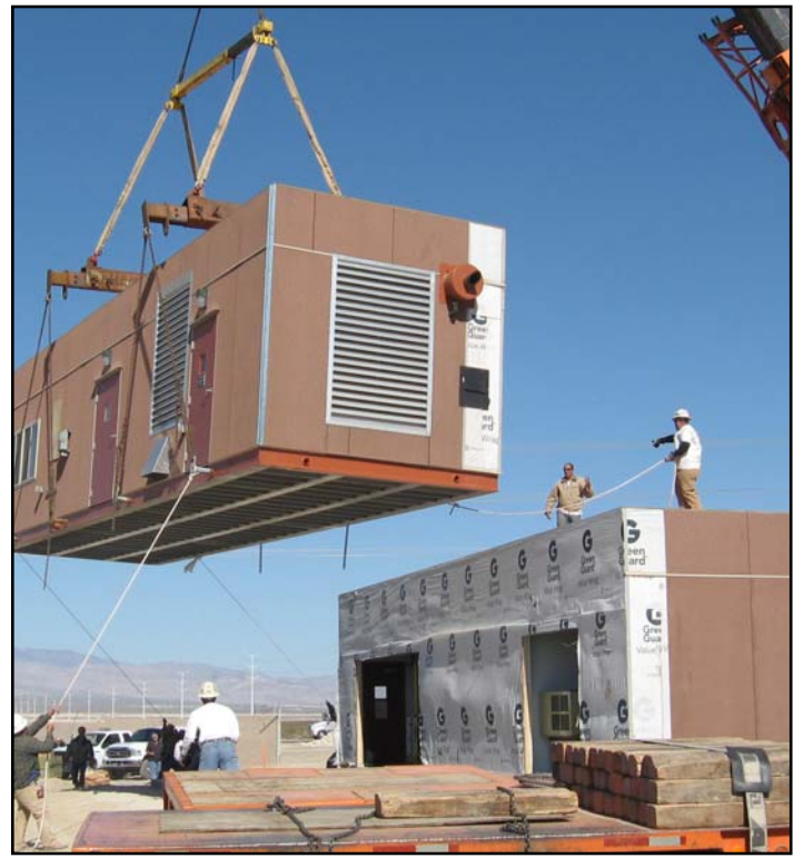
This project in Nevada is being installed side-by-side with its second half and has a desert colored ribwall exterior.
