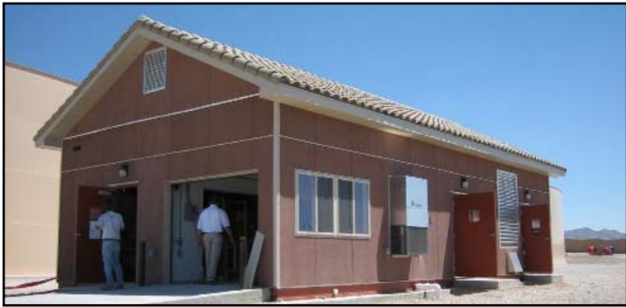
This is the finished Nevada project shown previously and has a roll up garage door and open/closing windows.
