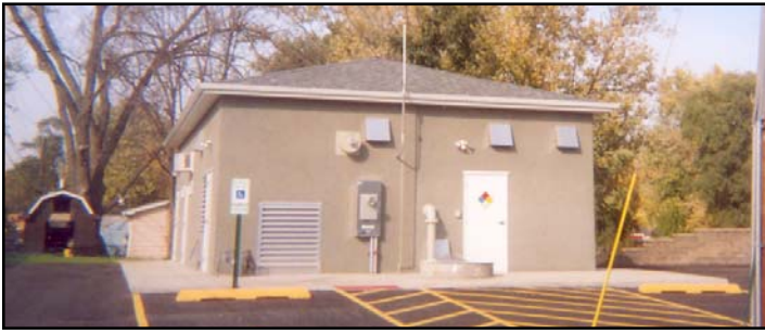
This project is located in Northern Illinois and has a factory-built water treatment system, new well houses, and a skid booster station with a fully integrated control and telemetry system.
