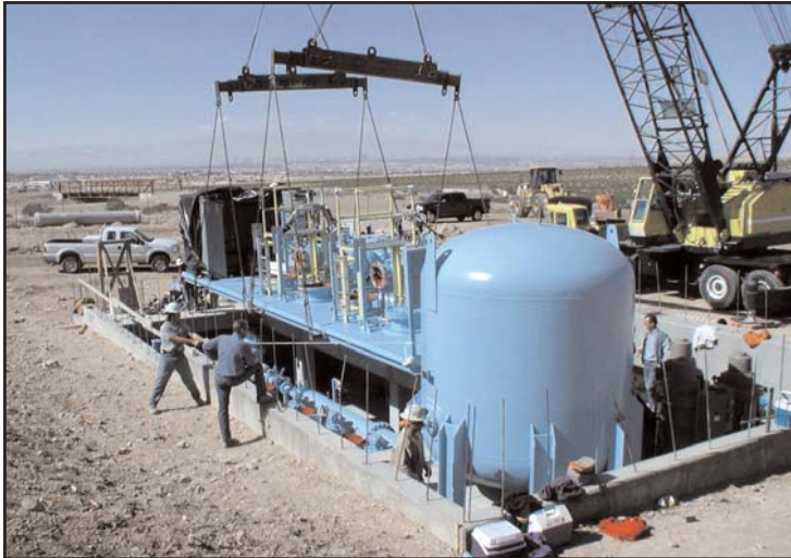
Skid being off-loaded and set into place with the 7500 surge tank.
