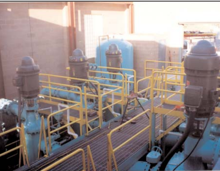
Assembled in building prior to adding roof.
