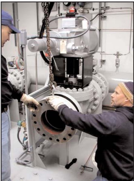
EFI pump installation crew.
